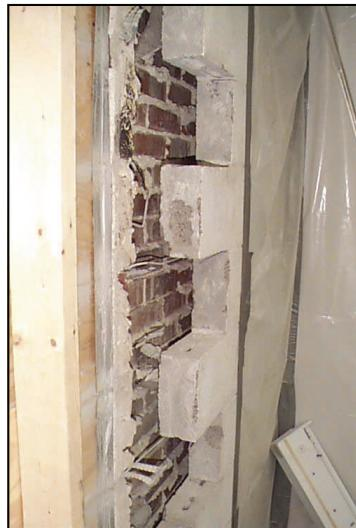
**Figure 3:** PCB remediation projects often include the removal of materials in contact with the PCB caulk due to unacceptable levels of residual PCB contamination.
