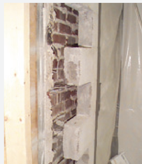
FIGURE 3 Brick and concrete block that absorbed PCBs from adjacent PCB-containing caulk has been removed from some buildings.
